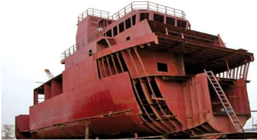
Hull Sections Being Assembled at Our Shipbuilding Yard
